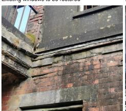
Steel beams to be retained and paired with new Existing chimney to be repaired and restored
