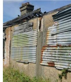
Defect Description: The existing steel/iron columns embedded in the external masonry walls are heavily corroded and are causing spalling of the surrounding concrete render.
