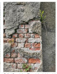
Defect Description: The existing brickwork is covered in cement render which is trapping moisture within the walls, leading to freeze thawweathering and would cause damp on internal finishes.
