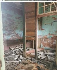
Timber and lead paint survey condition survey to be carried out. Timbers to be repaired and restored where possible.
